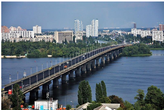
Figure 2: The longest entirely welded bridge (Paton bridge)
