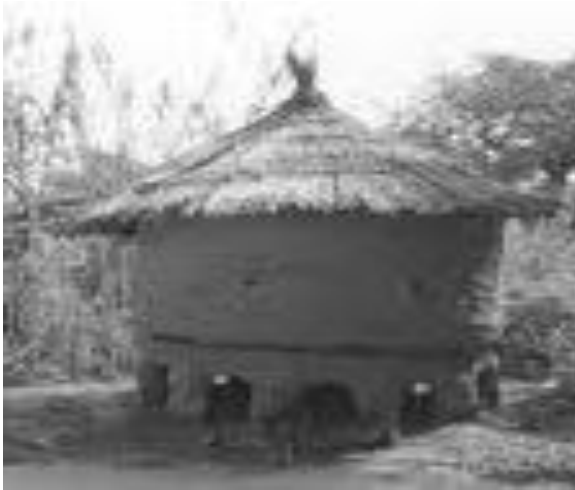
Plate 1. The mud silo similar to the one I was trained with at childhood
