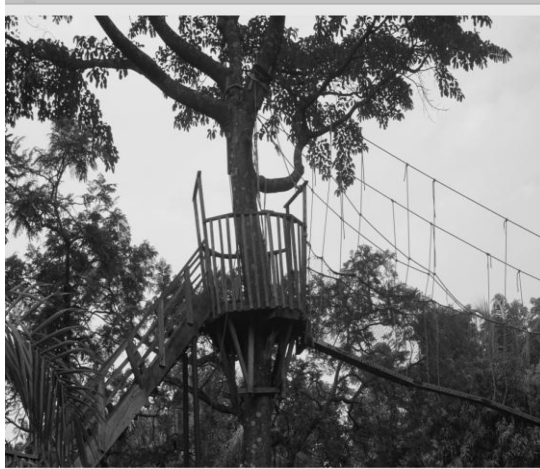
Plate 3b: The completed suspended walkway supervised by me in 2012
