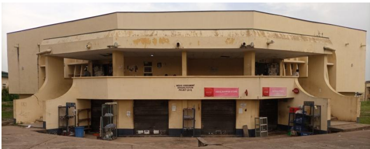
Plate 2a: The Lecture Theatre Science-Construction Supervised by me in 1997
